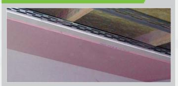
Hush bars are used to optimise acoustic performance by virtually decoupling a ceiling or wall lining from it's structure. This significantly reduces sound transmission through the floor, ceiling and wall structures. The Hush-Bar Deep resilient bar creates a larger void within a construction and allows high mass boards to be used. The Hush-Bar Deep can provide enhanced acoustic performance compared to standard resilient bars when used with a recommended lining.
