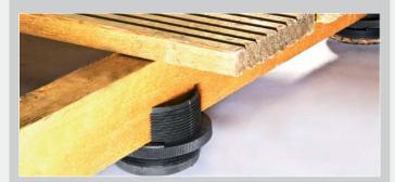
Hush Acoustic Decking Cradles are used to create a unique self levelling support system for decking areas.
