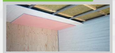
Hush Bar resilient bars are used to optimise acoustic performance by virtually decoupling a lining from a ceiling or wall structure. By using the Hush-Bars the airborne and impact sound transmission is significantly reduced. The Hush-Bars are one of the most important elements of a system to ensure compliance with the Building Regulations for sound transmission through separating ceilings and walls.
