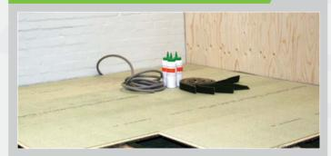
Hush-Panel 28 has been designed as a versatile impact reducing floor panel that can be used as a structural or an overlay board.
