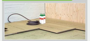
Hush-Panel 32 has been designed as an impact reducing floor panel, with added rigidity, that can be used as a structural or an overlay board. When used as a structural floor the stiffness of the upper layer accommodates wider joist centres, up to 600mm. A combination of the increase in mass and the Hushfelt™ resilient layer can produce superior results when used as part of a sound insulation system for separating floors.
