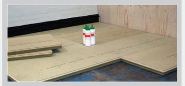
Hush Panel 52 has been designed specifically to combine two core components, required to comply with Robust Details FFT4 over concrete and steel and as an alternative floating floor solution to the traditional FFT-1 floor finish in timber frame development.
